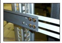
Fasten the Extension Bracket to the rear Outer Rail using 4 pcs M4x6 screws + Star Nuts. Adjust the post position, so outer rail will not take up any space between the left and right posts. Extension brackets can also be mounted to reach forward for shorter cabinets.
